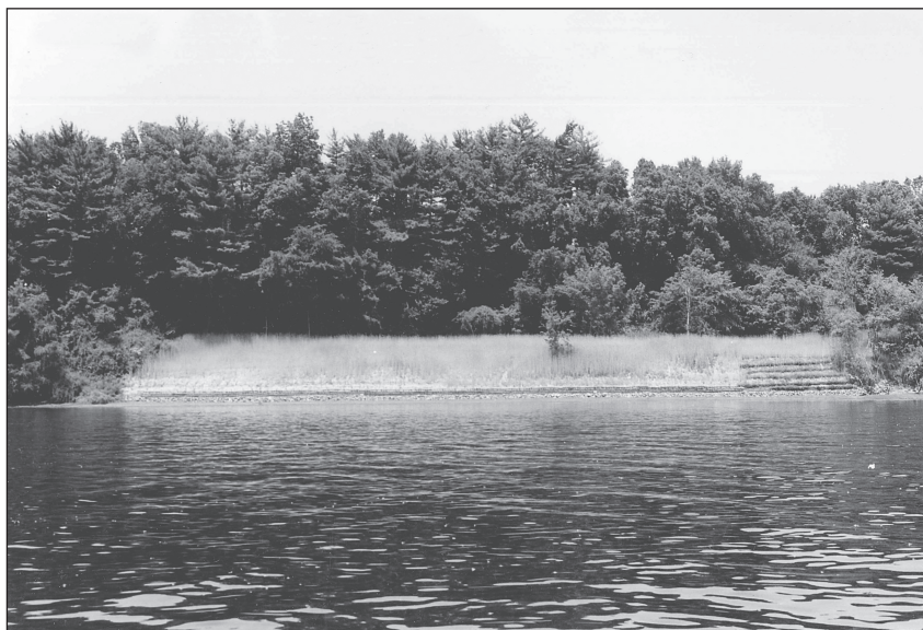
Figure 5. Stabilized bank. Current stabilization efforts in the Turners Falls Pool are done using a method called “bioengineering”; the banks are graded, creating a shallow slope, and a stone toe is installed. The bank is then covered with “fabric” and further stabilized with plantings.
